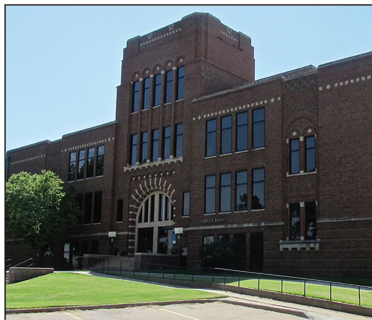
Jesse Dunn now stands where the castle once did. The front doors of Jesse Dunn face College street, where the front entrance of the castle was. Jesse Dunn was built during the great depression and was a part of a government project to create jobs. It, along with two other buildings, were constructed in 1937. Many people comment on the crazy architecture of Jesse Dunn, which was just the style that the architect was going for at the time. / Photo provided
