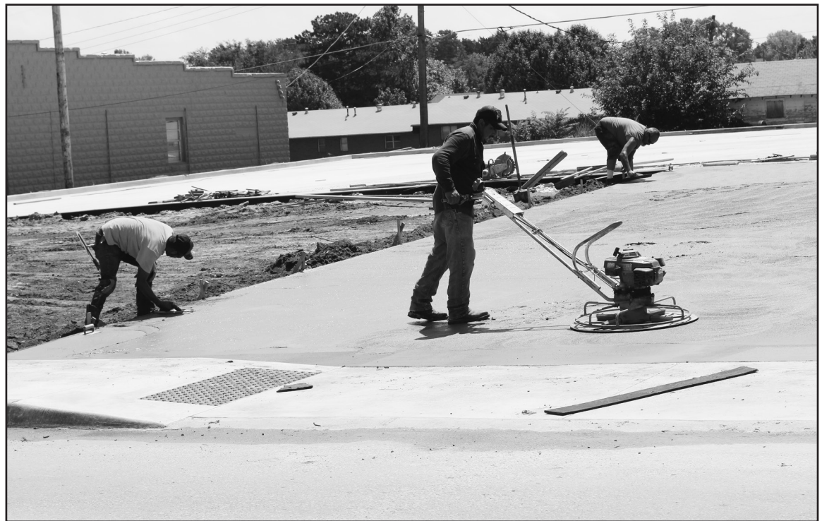
Workers pour concrete on the east gravel parking lot of South Hall on Aug. 16. /Photo by Kaylene Armstrong
