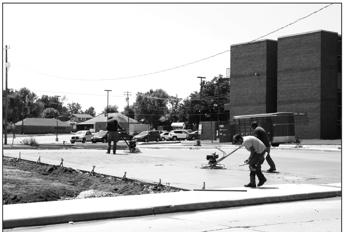
The money generated by students' parking fees helped fund the renovation of just one South Hall's parking lots. Now both of South Hall's parking areas are paved. /Photo by Kaylene Armstrong
