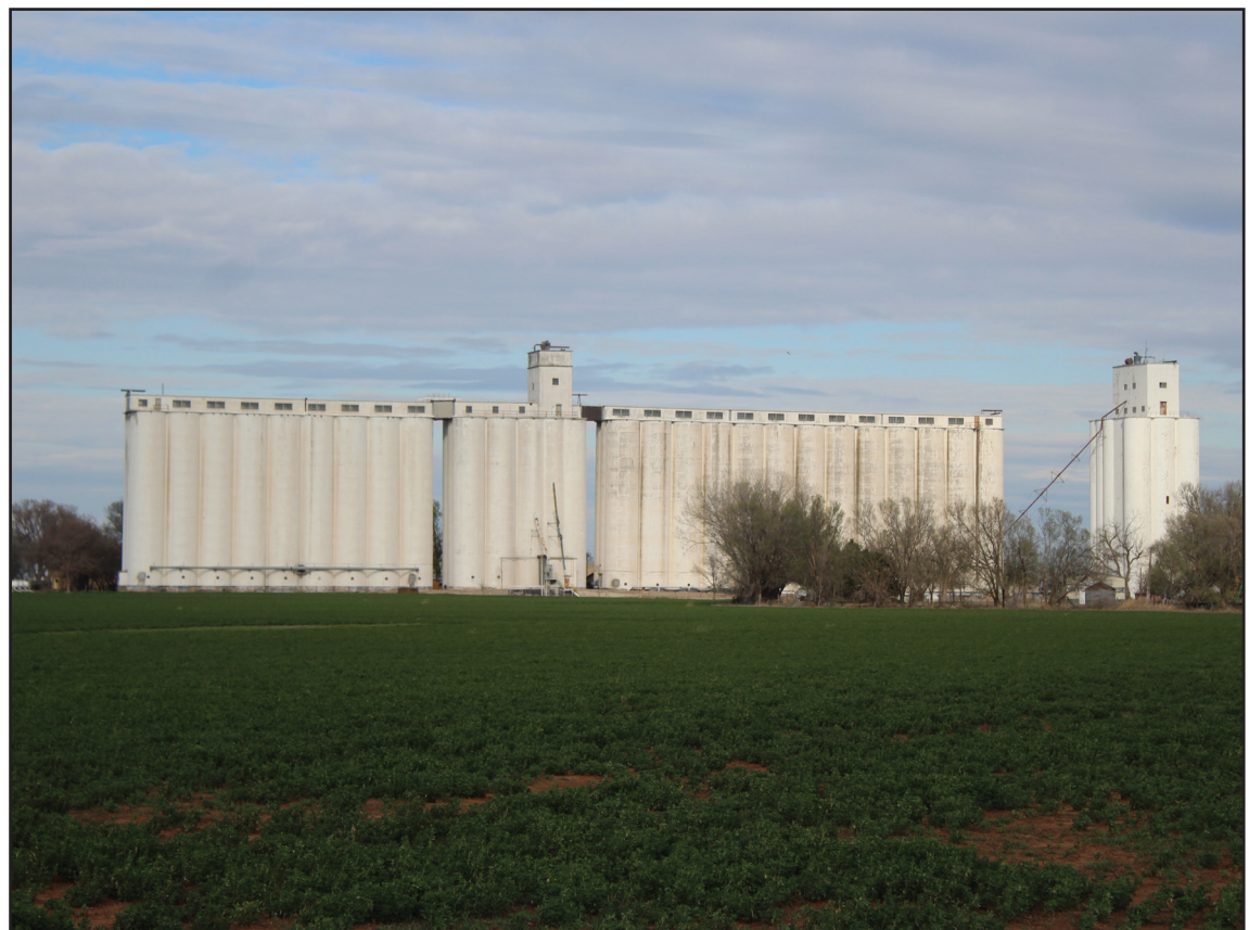
A picture perfect view of the grain elevators in Burlington, OK.
