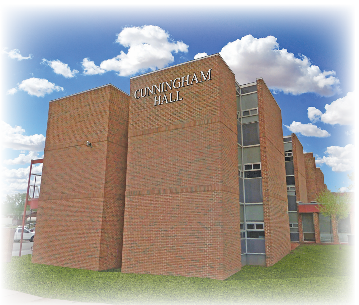
Photo provided by Easley Associates Architects
