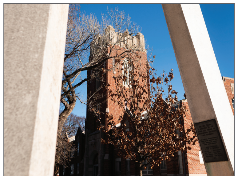
A look at Herod Hall now through the supports of the bell tower. The bricks underneath the tower supports came from the Castle on the Hill after fire destroyed it March 1, 1935. Photo by Ingrid Maldonado
